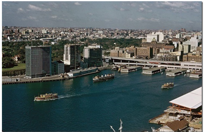
Circular Quay 1960 - the Overseas Terminal under construction on the right
